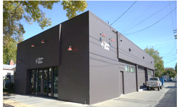
Uptown Studios converted an old warehouse space into a modern, energy efficient workplace.
