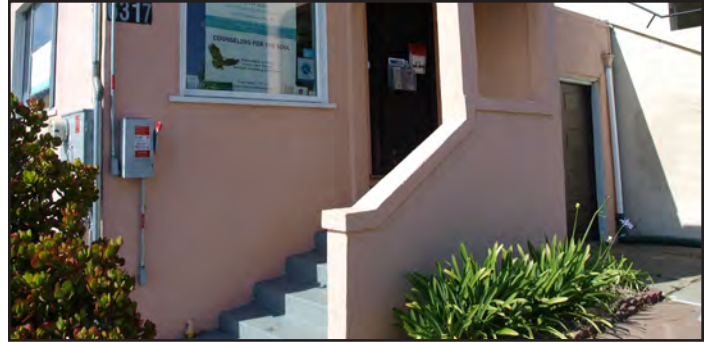
Street View of Transformative Wealth Management's Historical and Green Office Building (with drought friendly landscaping too!).
