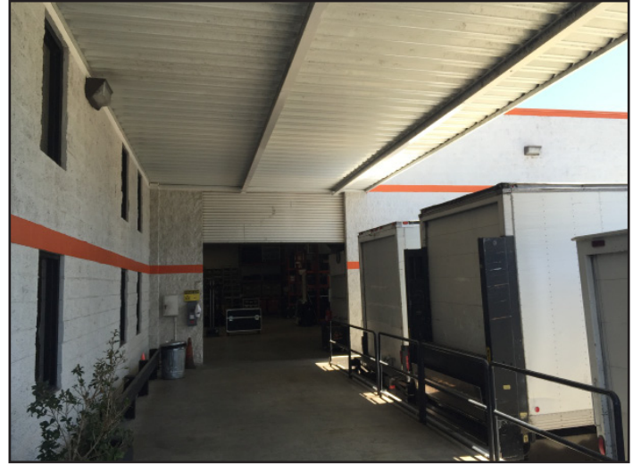
LED lights were installed in the loading dock of ShowPro's parking lot.
