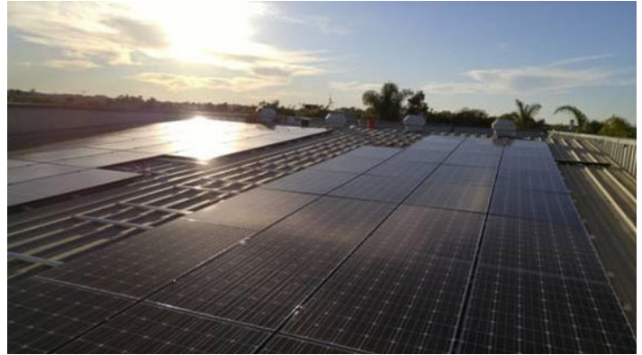
The headquarters of Santa Barbara Airbus gathers most of its electric power needs from the 134 solar panels installed on the rooftops.
