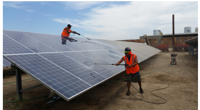
Mr. Squeegee's team cleaning a solar panel array in an agriculture community.
