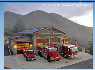
Marin County's Throckmorton fire station is LEED-Gold certified and includes a 38 kilowatt photovoltaic system, renewable and recycled content building materials, low-emitting materials, and water efficient landscaping.
