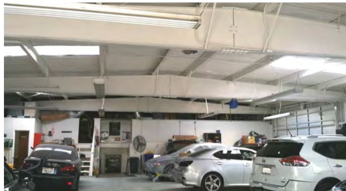
To add natural light and reduce electricity usage, skylights were added to the body shop repair area.
