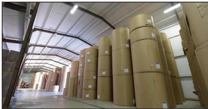
Warehouse uses energy efficient T8 lighting and motion sensors.
