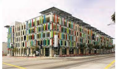
The nation's first sustainable, solar-powered parking structure is in Santa Monica. The six-story, 882-space structure at the Civic Center (shown above) features photovoltaic roof panels, a storm drain water treatment system, recycled construction materials and energy efficient mechanical systems.
