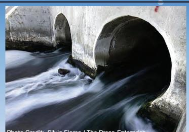
Photo Credit: Silvia Flores / The Press-Enterprise Treated water flows into a channel that will bring it to the Santa Ana River (shown above). Riverside's Recycle Water Project uses treated wastewater to irrigate City land.
