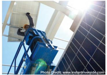
The Casa Blanca Library in Riverside was retrofitted with a new 54.88 kilowatt solar energy system (shown above) in April 2009. The system is affixed to the top of the Library's parking structure.
