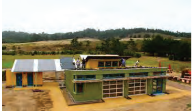
The Green Classroom under construction.
